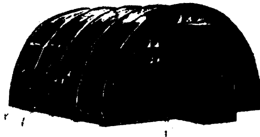
Figure 3-3. Tent, frame type, sectional.
